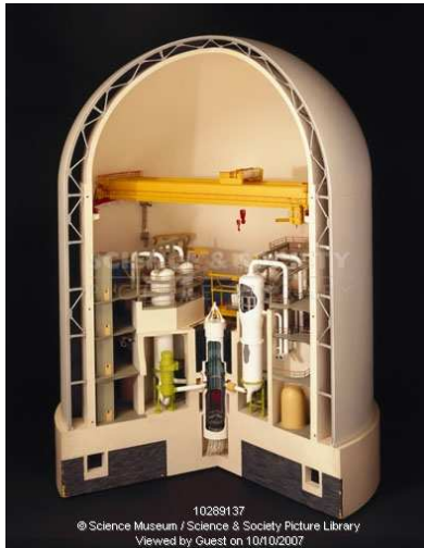
Figure 3.5 - Schematic of the Sizewell B PWR , commissioned in 1995. (Courtesy of ‘The Science & Society Picture Library’: http://www.scienceandsociety.co.uk/ )
