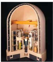
Figure 3.5 - Schematic of the Sizewell B PWR, commissioned in 1995. (Courtesy of 'The Science & Society Picture Library': http://www.scienceandsociety.co.uk/)
